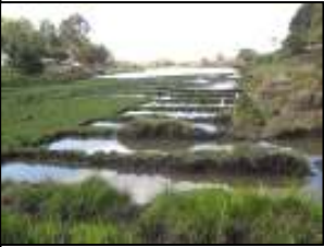
Work on Dam 1
