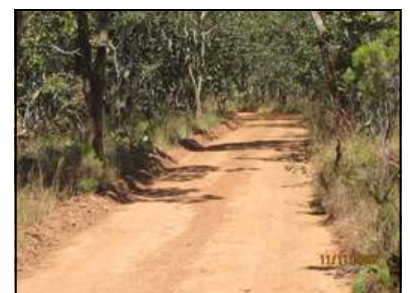
Runyina road after grade
