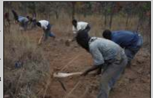
Road cutting at Lower Chelinda
